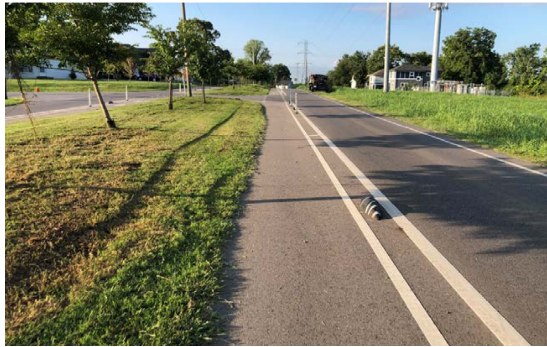
GROUND LEVEL PROTECTIVE BARRIERS
