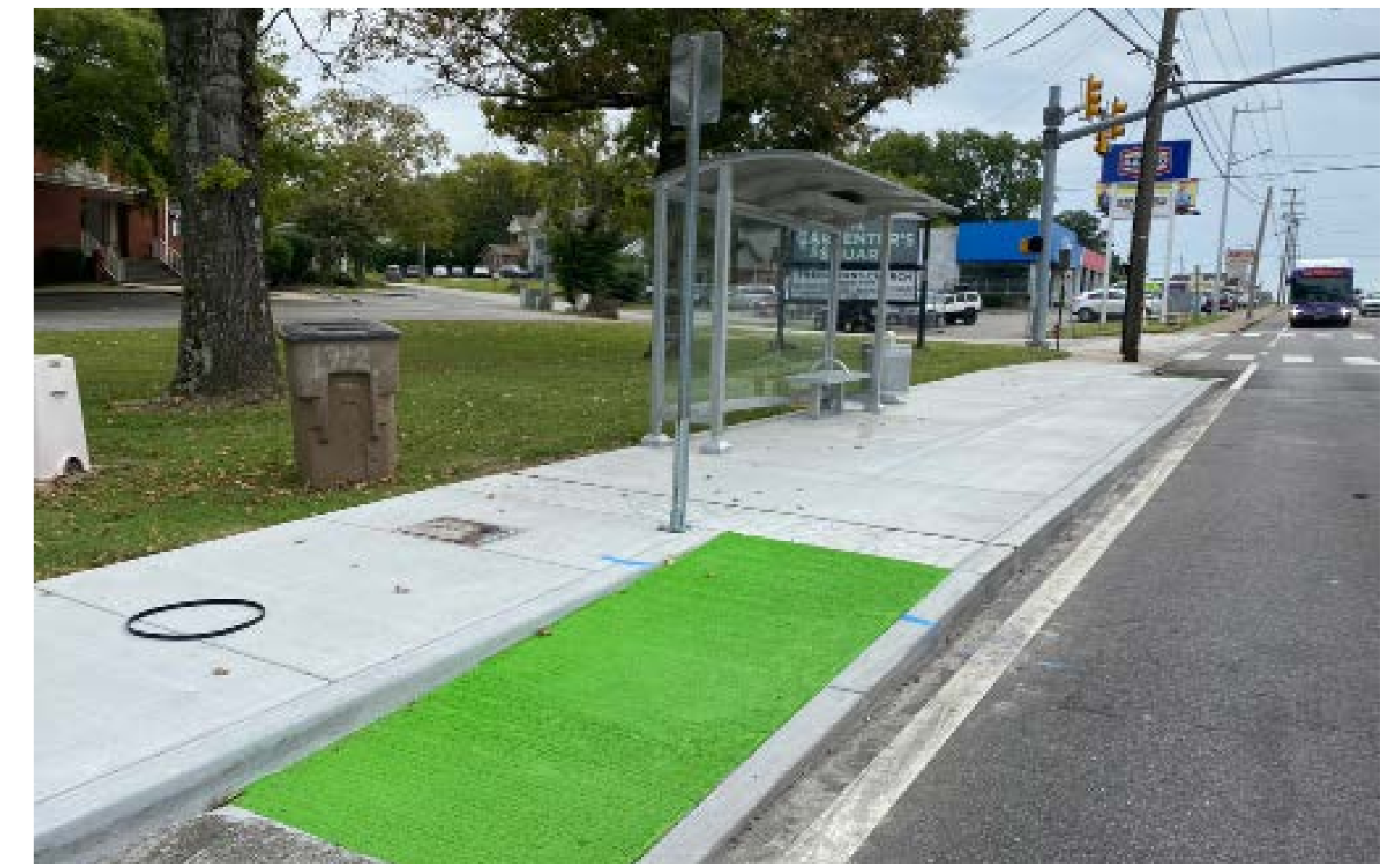
DESIGNATED BICYCLE LANE AND TRANSIT STOP
