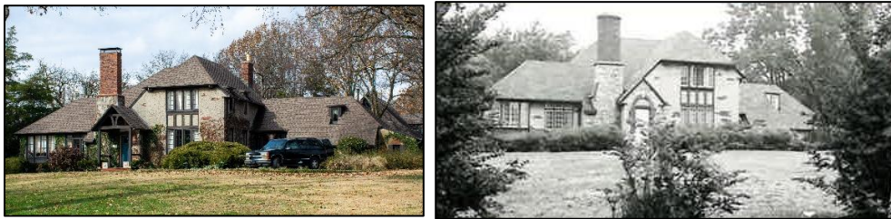
Figure 13: The house at 1637 S Observatory Dr as seen in 2024 (Metro Historical Commission) and 1969 (Property Assessor).
