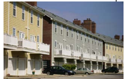
Rear access parking garages
