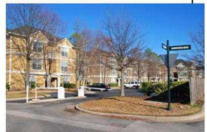
Landscaping and screening
