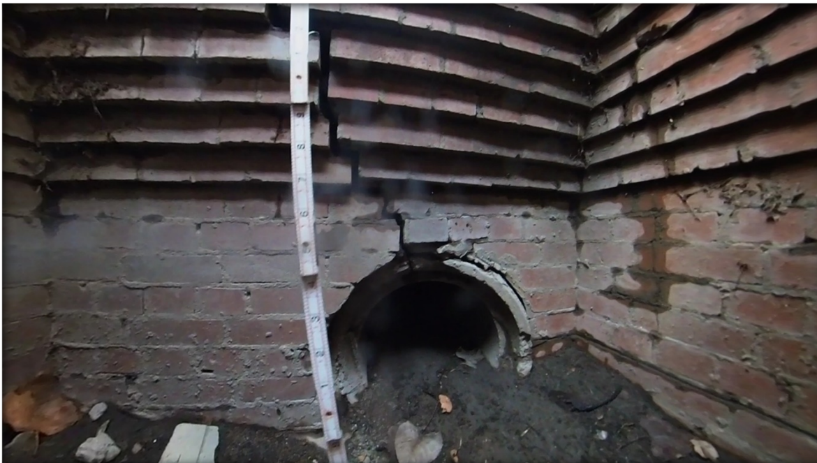
Figure 5.6 – Example of Grade 4 – Poor Condition (significant cracking, near failure)
