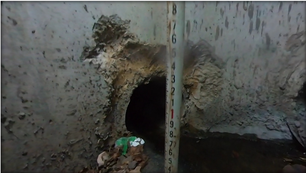
Figure 5.5 – Example of Grade 3 – Fair Condition (moderate defects, exposed aggregate)
