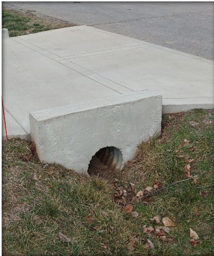
Figure 5.2 – Example of Grade 0 – Excellent Condition (new construction, no defects)
