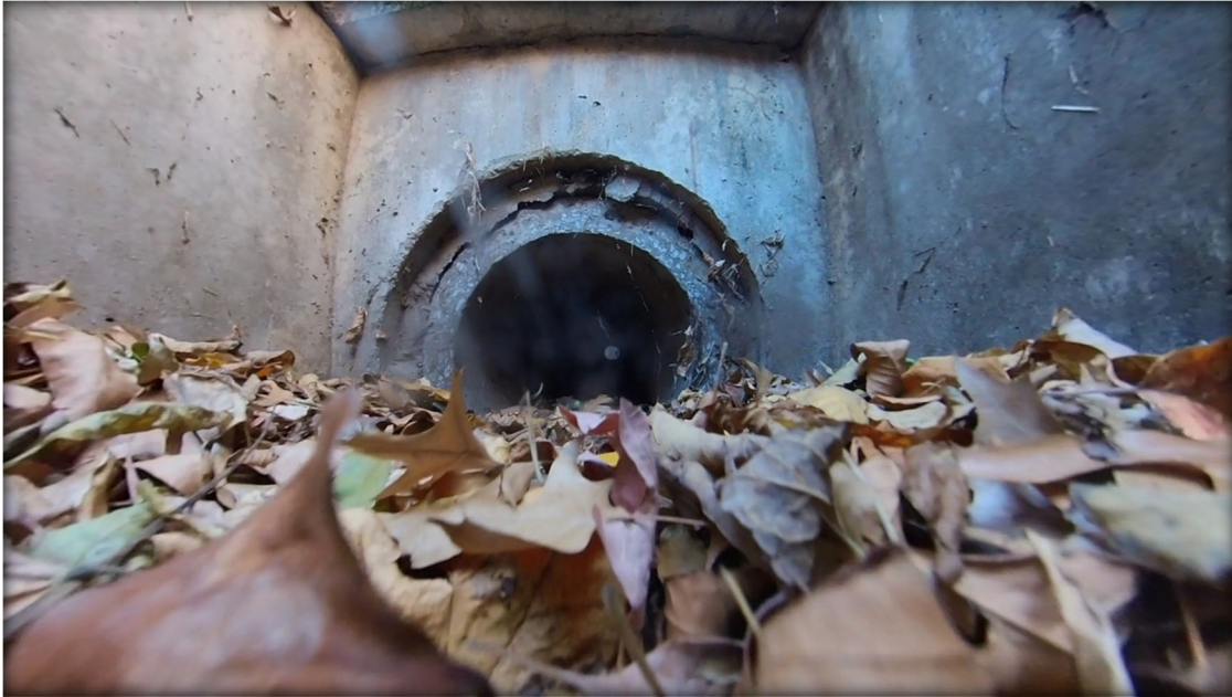
Figure 5.4 – Example of Grade 2 – Moderate Condition (several minor defects)
