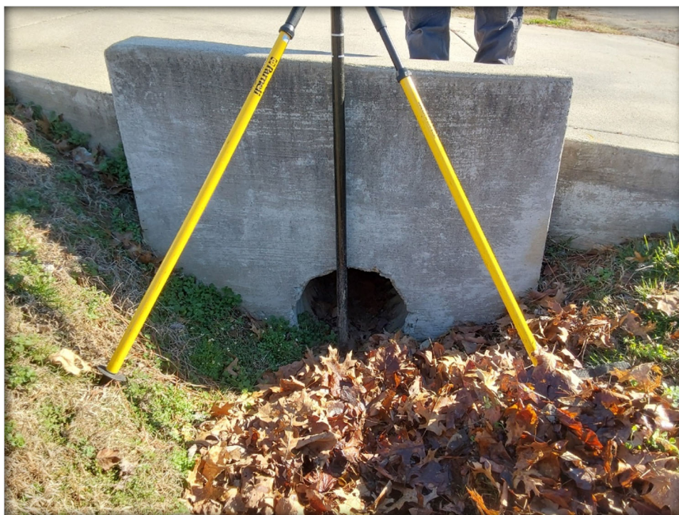
Figure 5.3 – Example of Grade 1 – Good Condition (minor defects, most of service life left)
