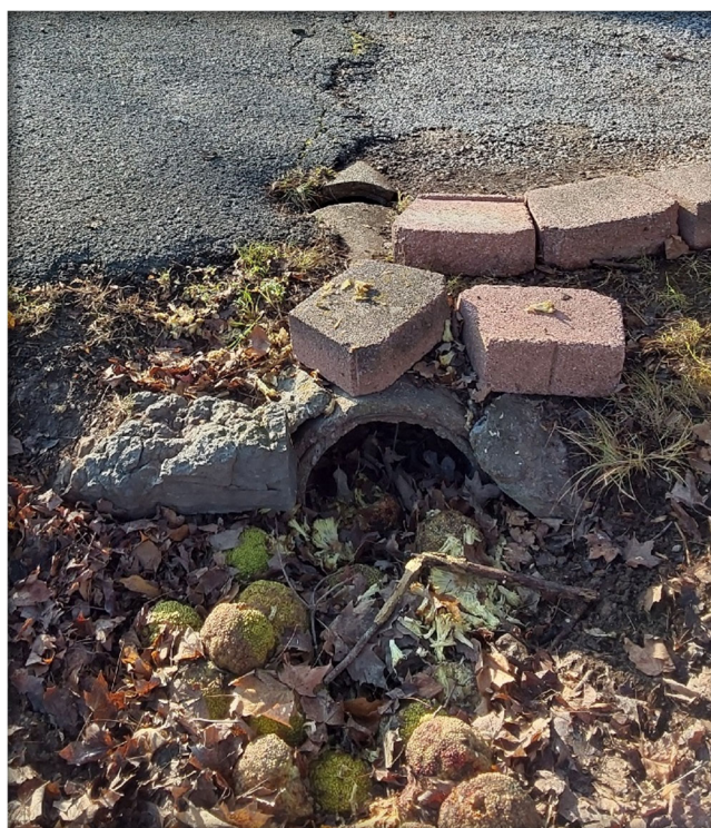
Figure 5.7 – Example of Grade 5 – Failed Condition (pipe completely separated)
