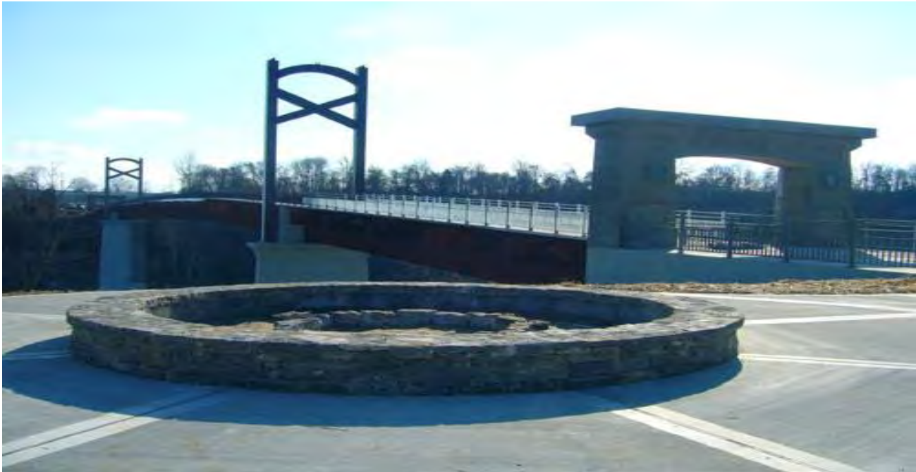
Cumberland River Pedestrian Bridge – Stones River Greenway
