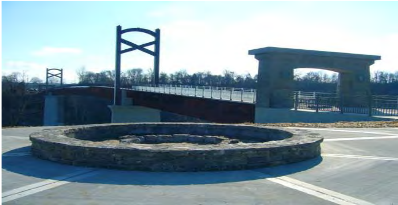
Cumberland River Pedestrian Bridge – Stones River Greenway
