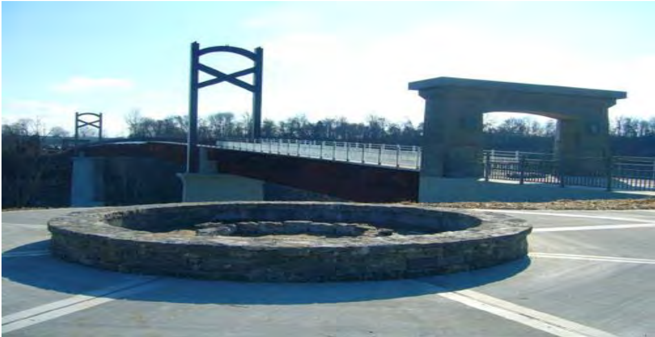
Cumberland River Pedestrian Bridge – Stones River Greenway
