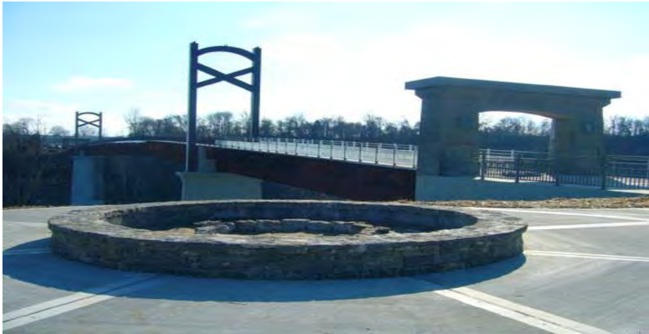
Cumberland River Pedestrian Bridge – Stones River Greenway
