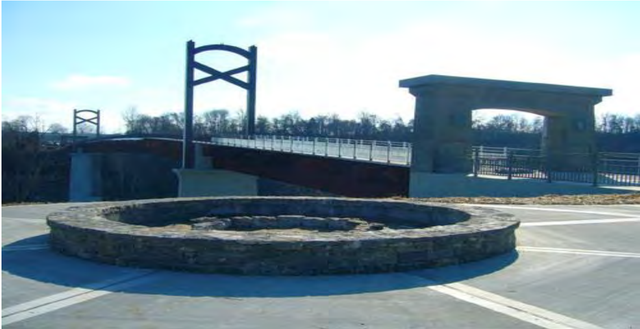
Cumberland River Pedestrian Bridge – Stones River Greenway
