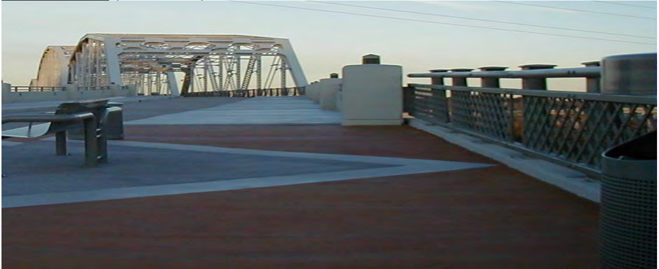
Shelby Street Bridge Walkway
