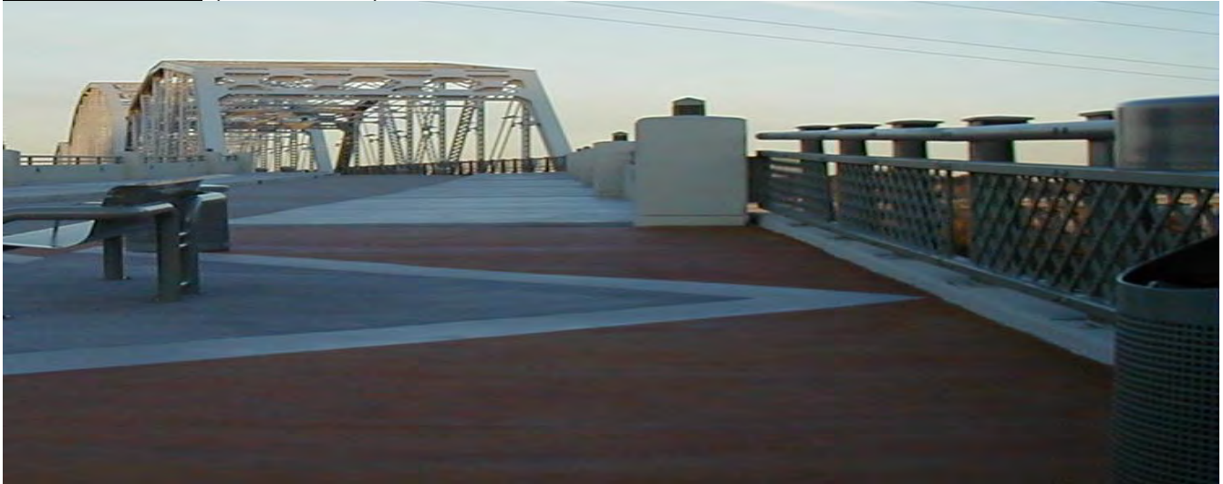
Shelby Street Bridge Walkway
