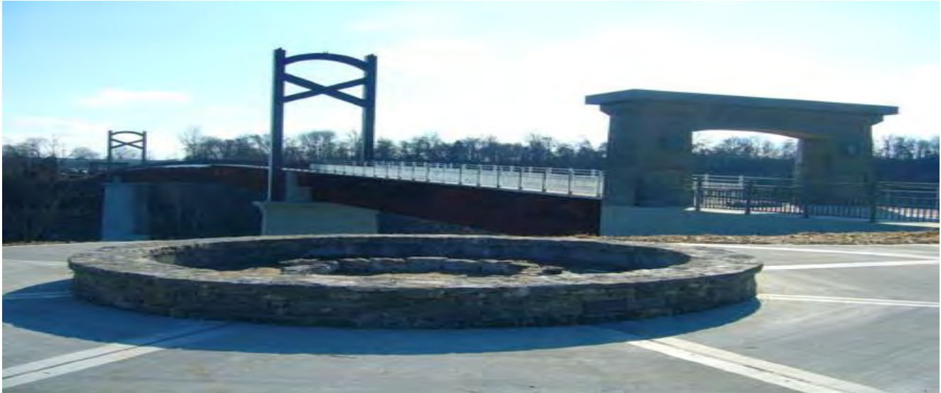
Cumberland River Pedestrian Bridge – Stones River Greenway
