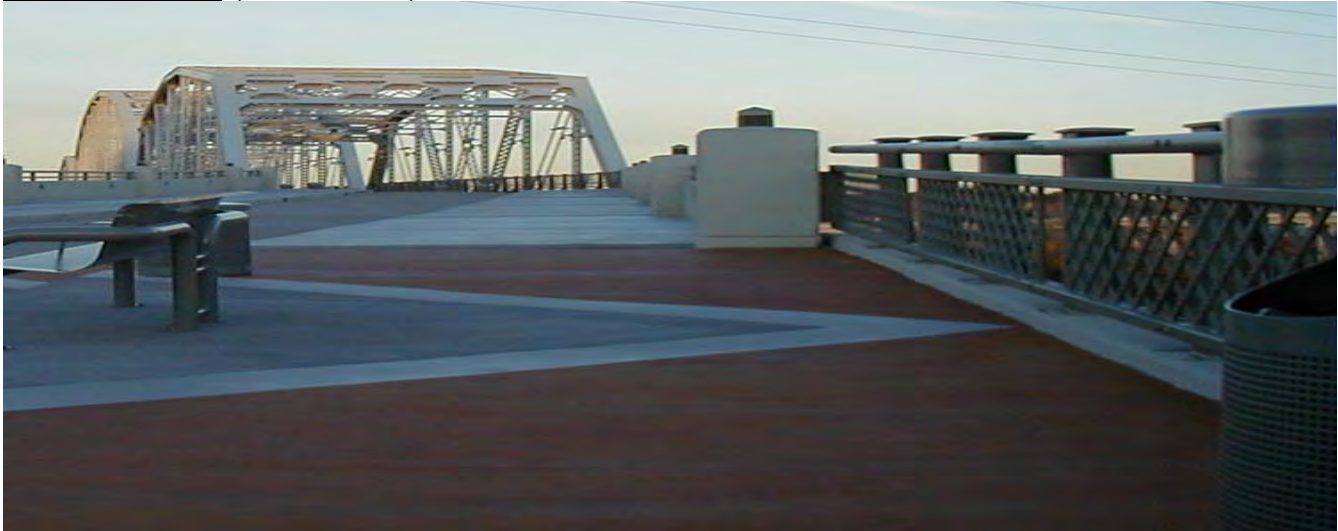
Shelby Street Bridge Walkway
