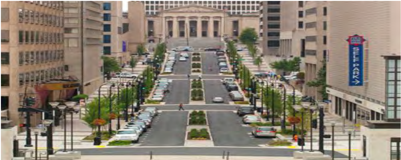
Deaderick Streetscape Improvement Project
