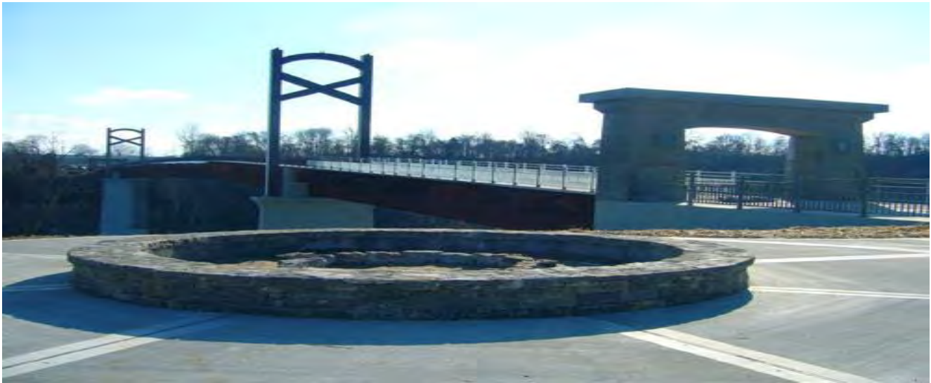
Cumberland River Pedestrian Bridge – Stones River Greenway
