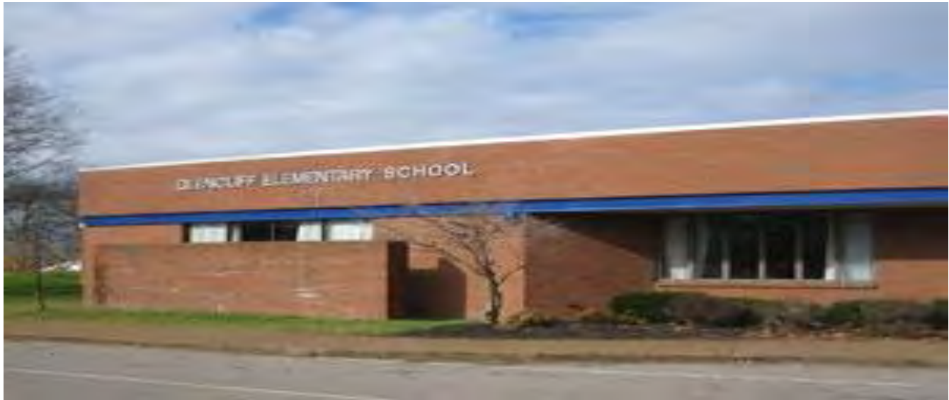
Glenclyff Elementary School
