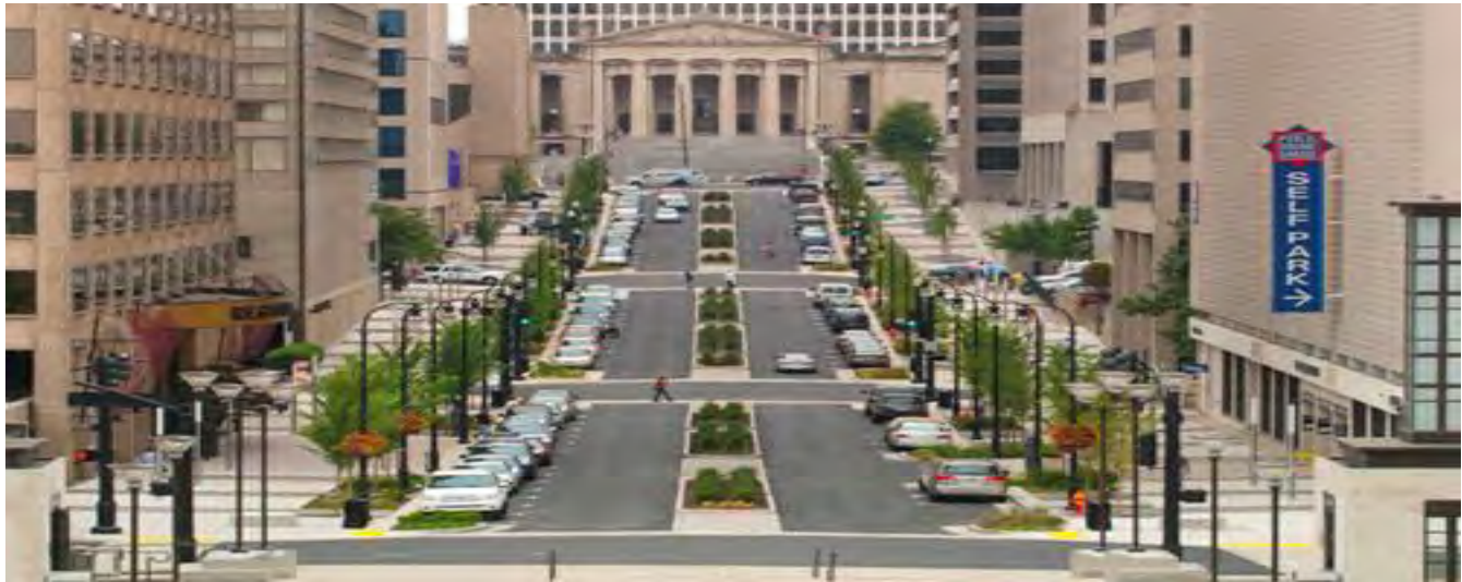
Deaderick Streetscape Improvement Project
