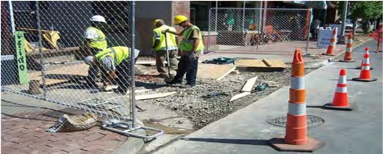
Intersection / Sidewalk Re-Construction – 21 st Avenue
