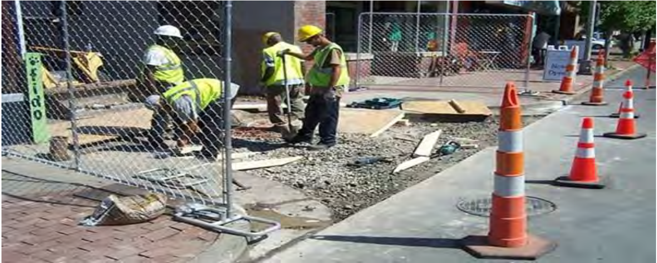
Intersection / Sidewalk Re-Construction – 21 st Avenue
