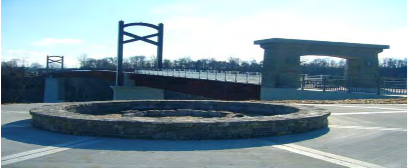
Cumberland River Pedestrian Bridge – Stones River Greenway
