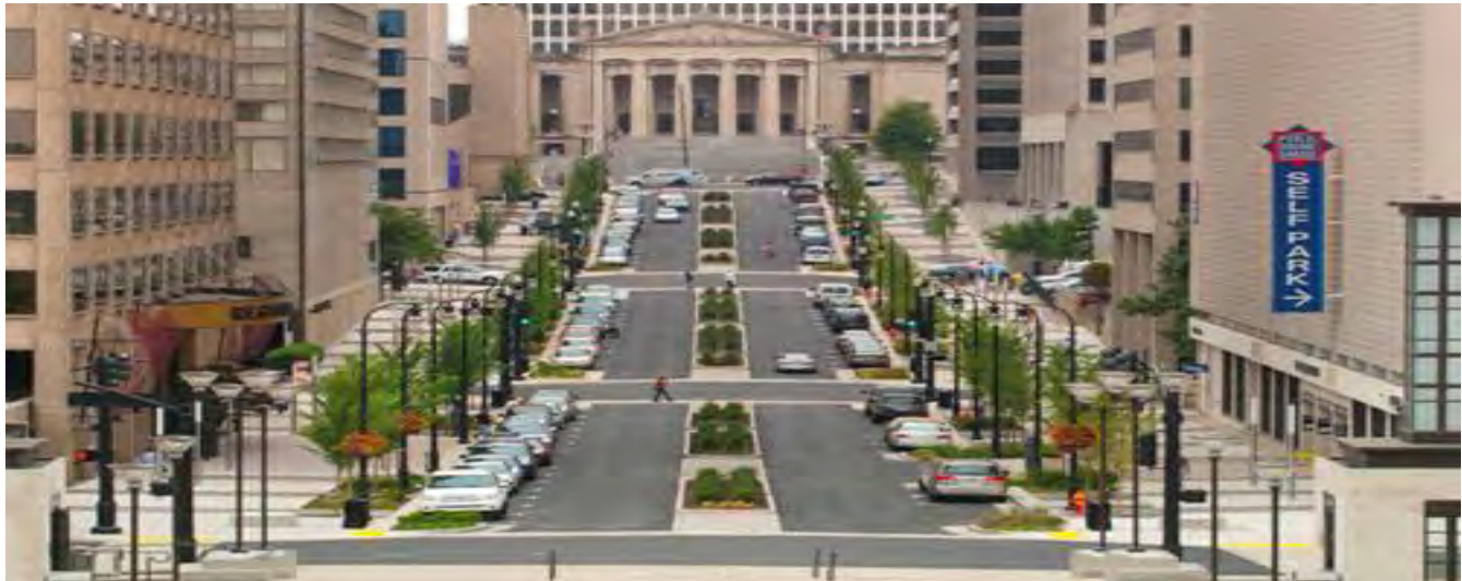
Deaderick Streetscape Improvement Project
