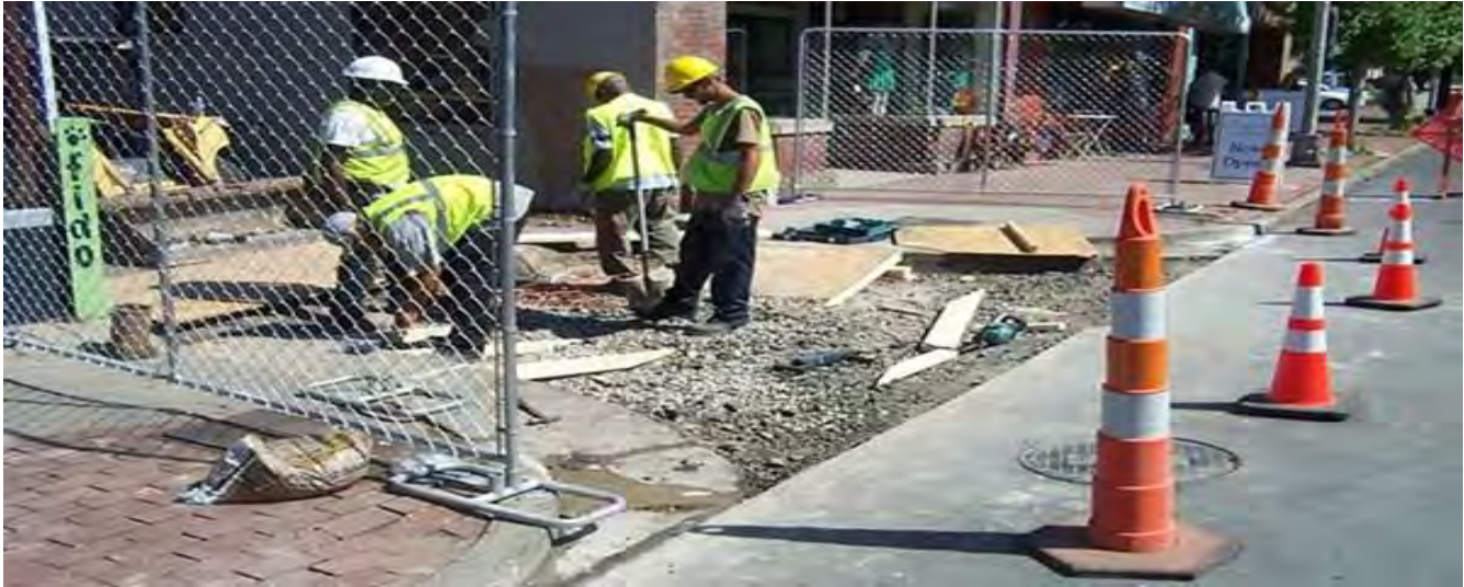
Intersection / Sidewalk Re-Construction – 21 st Avenue
