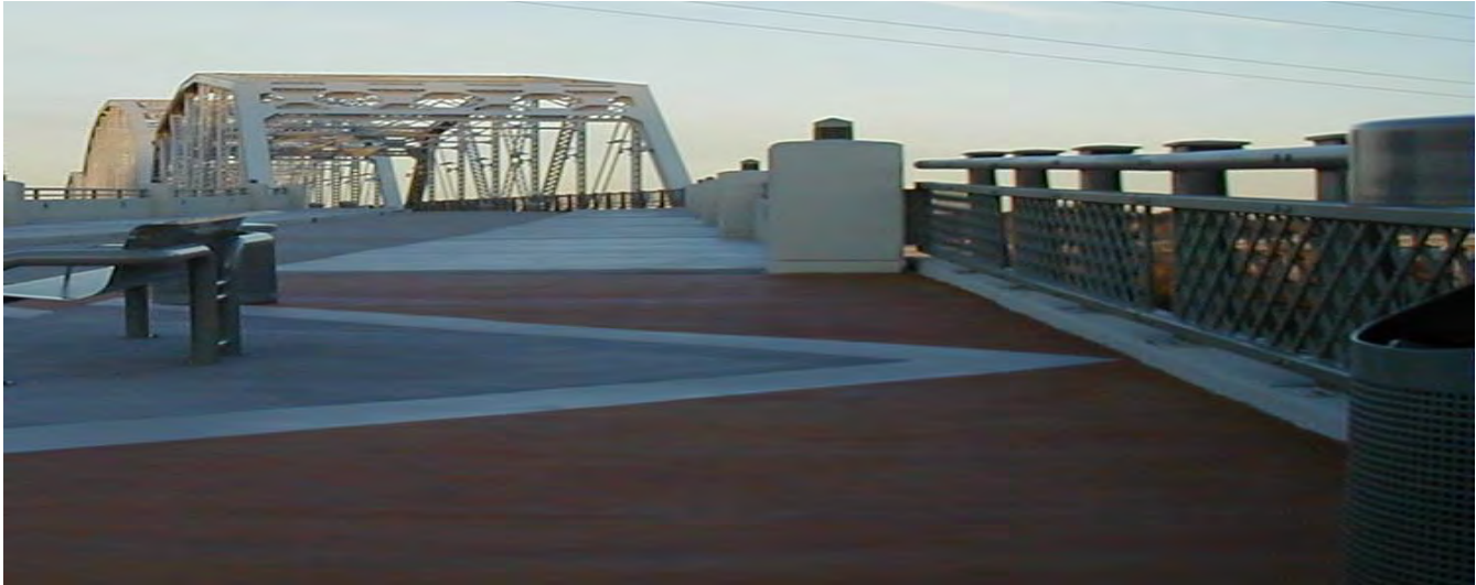
Shelby Street Bridge Walkway
