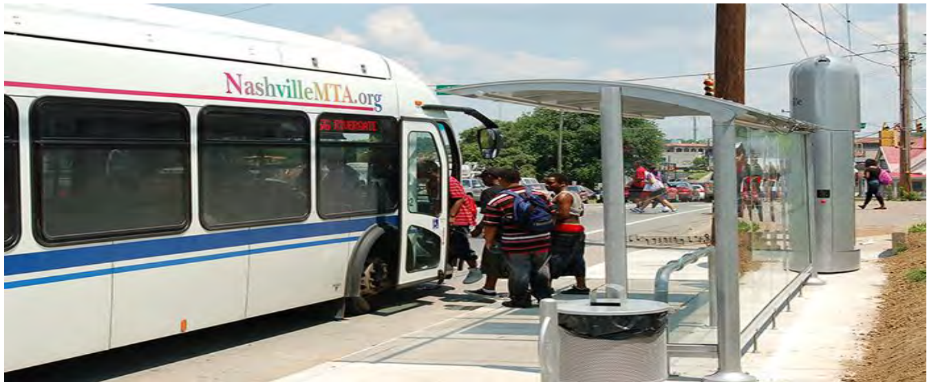
MTA's Bus Rapid Transit (BRT) Gallatin Road
