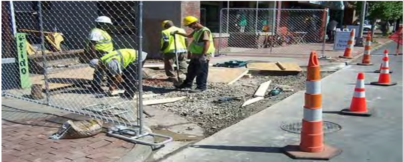
Intersection / Sidewalk Re-Construction – 21 st Avenue
