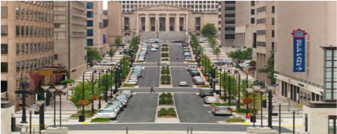
Deaderick Streetscape Improvement Project
