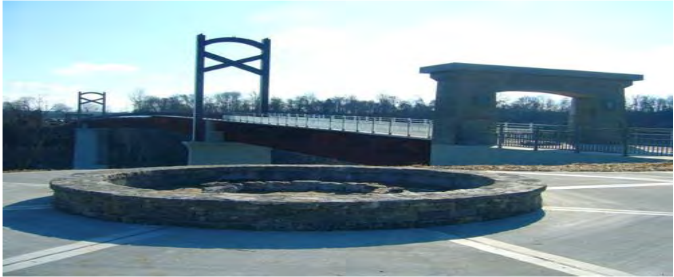
Cumberland River Pedestrian Bridge – Stones River Greenway
