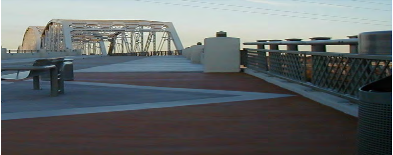
Shelby Street Bridge Walkway
