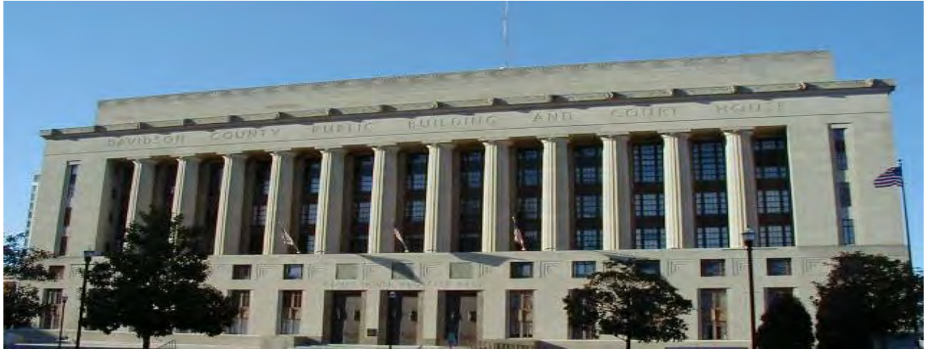
Historic Nashville Metro Courthouse
