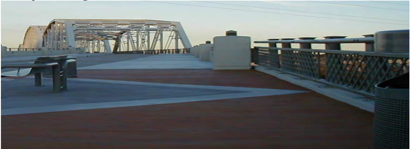
Shelby Street Bridge Walkway
