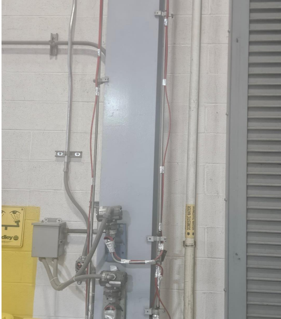
Heat Trace on Steam Pressure Transmitter
