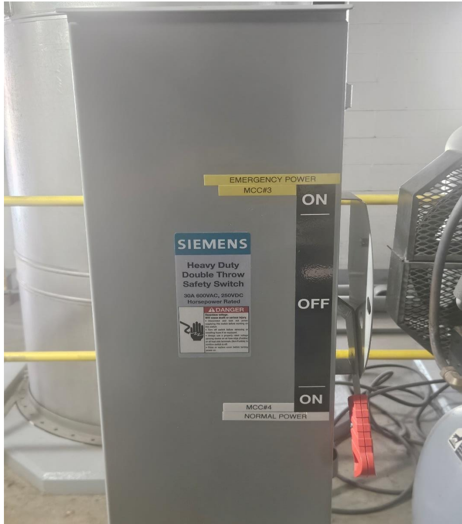
Plant Control Air Compressor Transfer Switch
