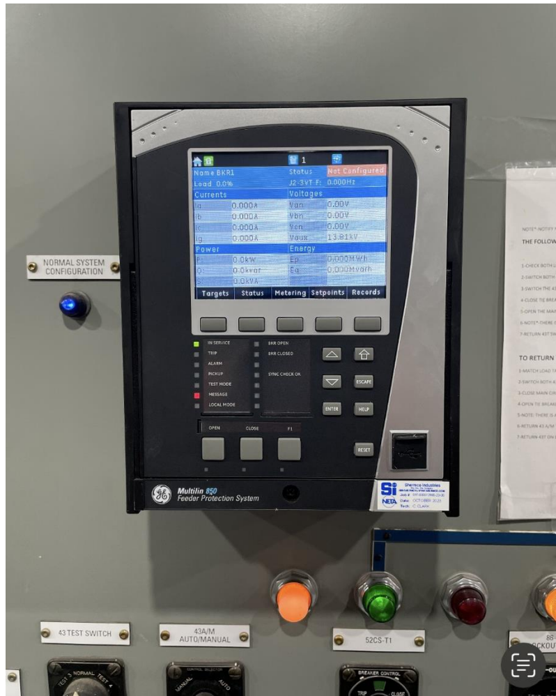
Upgraded Tie Breaker Relay between SWGR 1A and SWGR 1B
