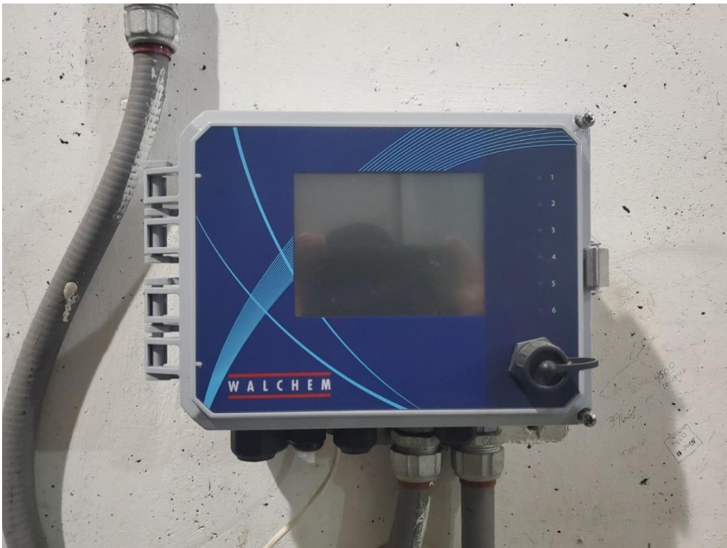
Boiler #4 Blowdown Controller (New Panel)
