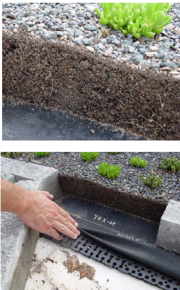
Figure 12.1. Photos of Vegetated Roof Cross-Sections (source: B. Hunt, NCSU)
