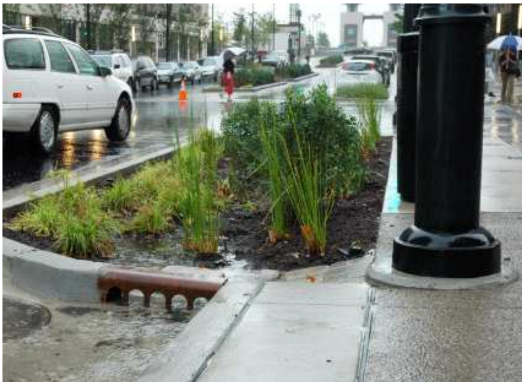
Figure 4.5—Existing Bioretention Areas Along Deaderick Street.
