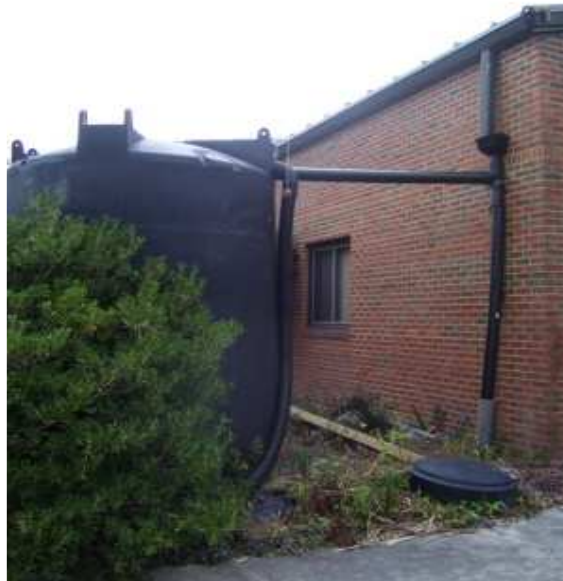
Rainwater Cistern Source: Craven County, NC
