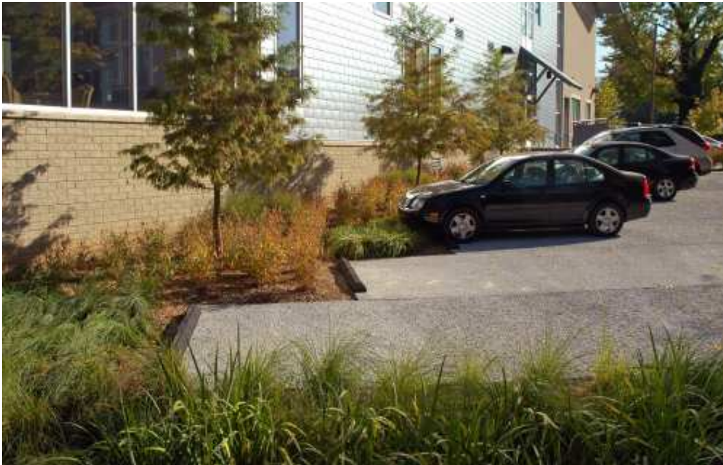
Figure 4.4—Existing Pervious Concrete Parking at TN Association of Realtors.
