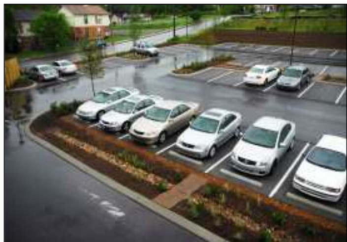
Figure 3.33—1700 Charlotte Ave. Bioretention.
