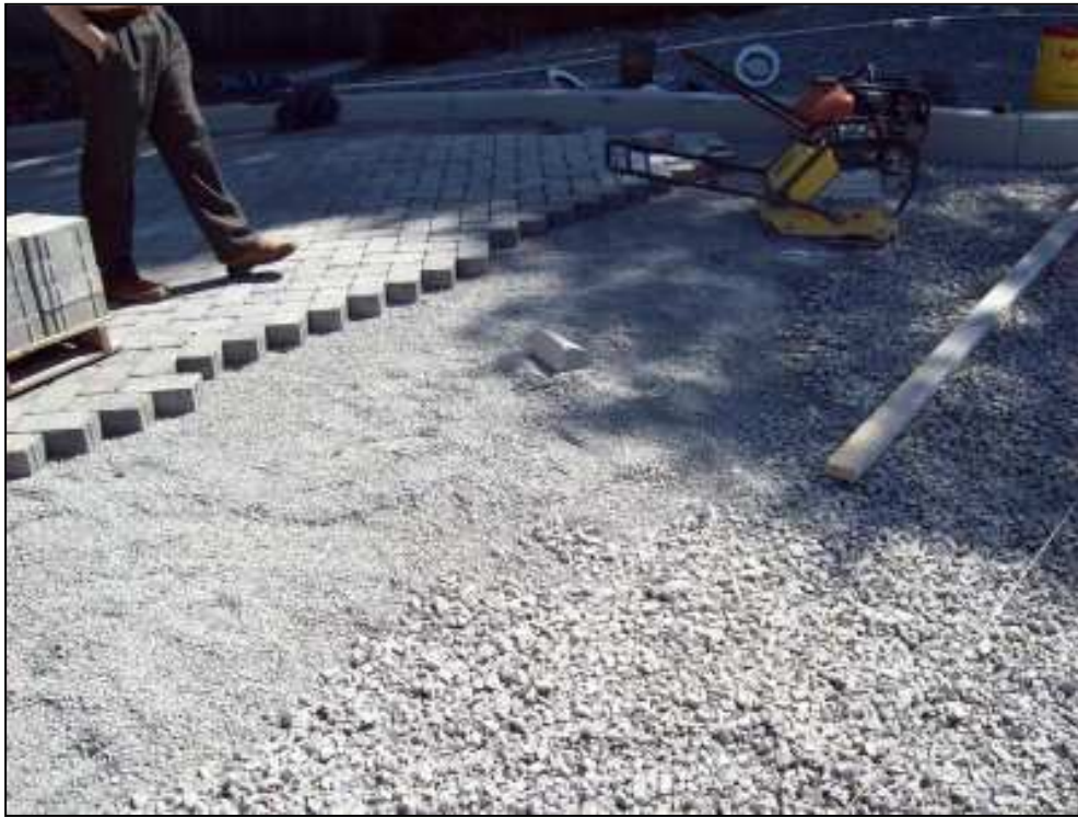
Figure 3.37--Permeable Paver Construction St. Johns Church, Knoxville.
