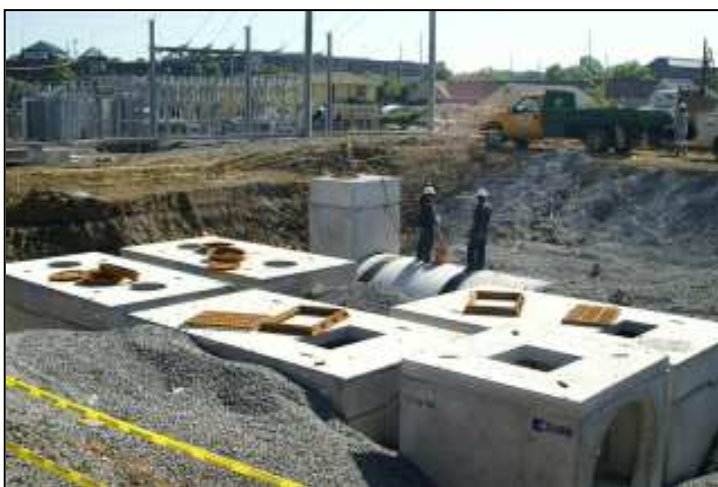
Figure 3.8—Example of Underground Cistern.
