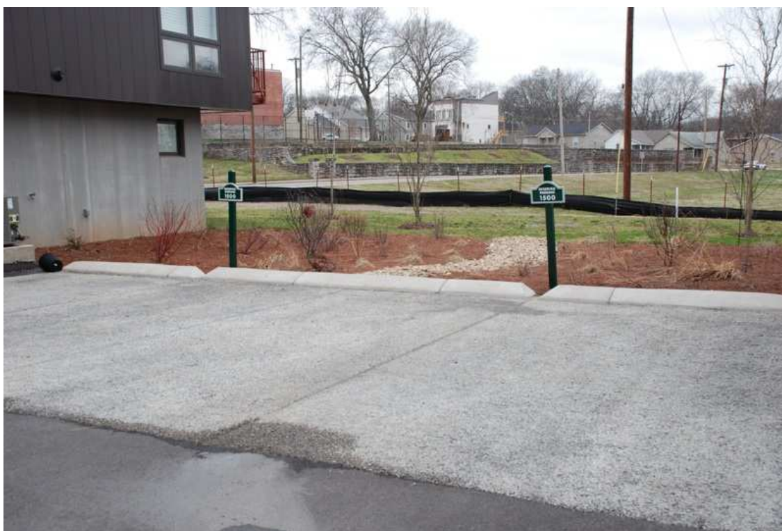
Figure 4.3—Porous concrete and Bioretention Area at Morgan Park Place.
