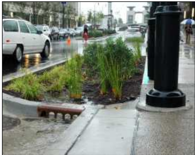
Figure 3.32--Bioretention at Deaderick St.
