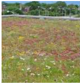
Extensive Green Roof
