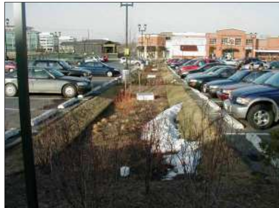
Bioinfiltration Source: LID Center
