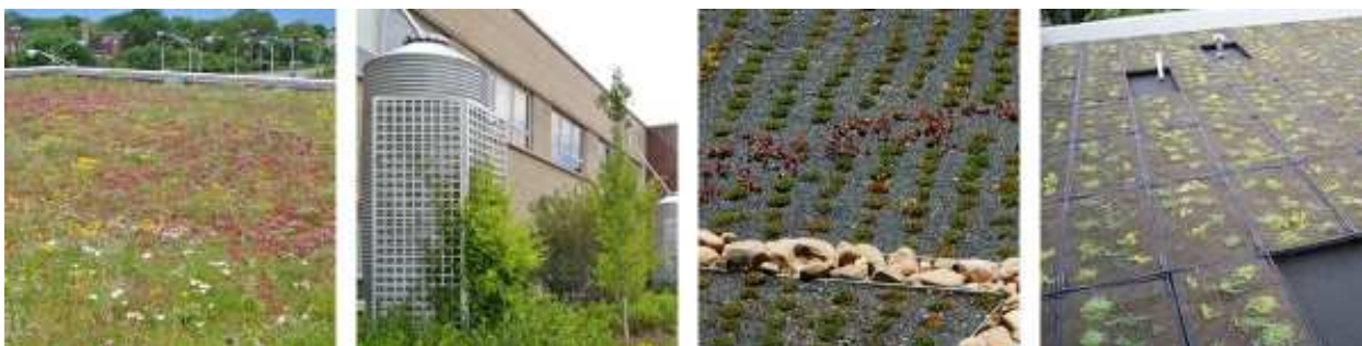
Extensive Green Roof
