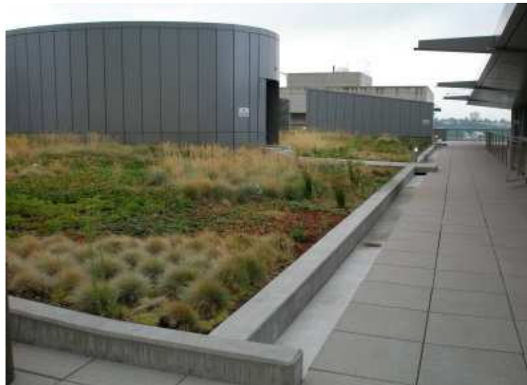
Seattle City Hall Green Roof Source: SvR Design Company
