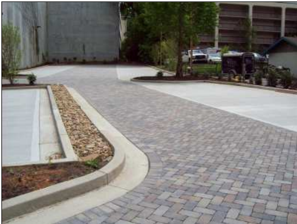
Figure 3.38--Permeable Pavers Gatlinburg Hilton Hotel.
