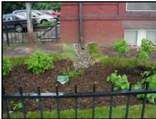
Downspout Disconnection into Vegetated Area Source: LID Center
