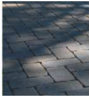
Pervious Concrete Pavers
