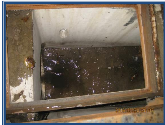
Photographs of the Polymer Spill onto the MS4
