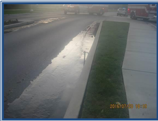
Photographs of the Polymer Spill onto the MS4
