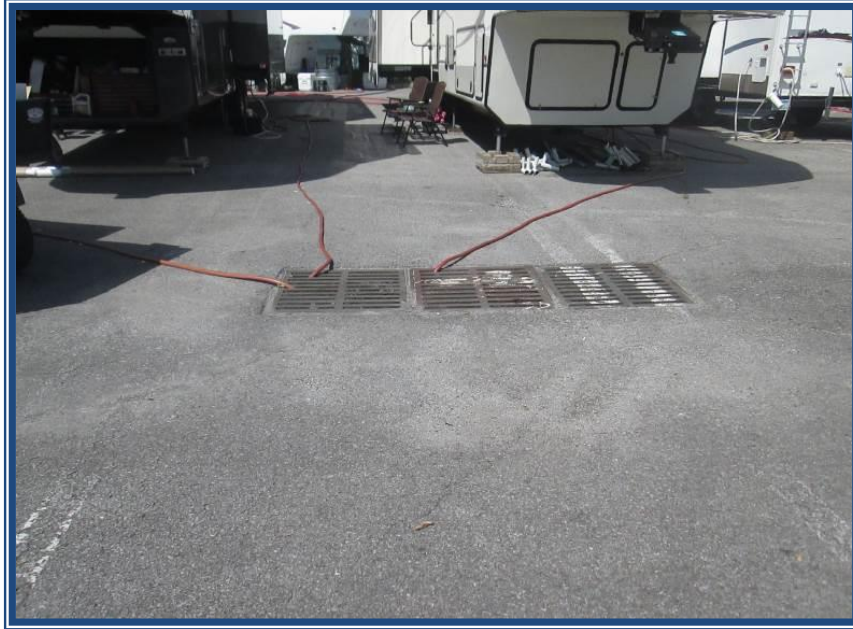
Discharge of Gray water from the Travel Trailer
