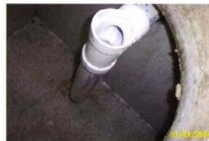
**Proper Outlet T installation**
