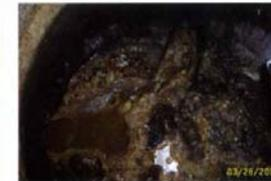
Fats, Oils & Grease (FOG) discharge from a food service establishment causes blockages in sewer lines, which result in sanitary sewer overflows.
