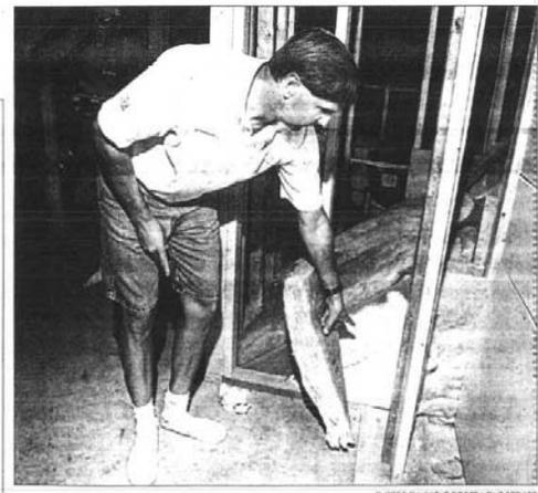
Homebuilder John Harris pulls back insulation to reveal spray-in foam insulation used to create a tighter more efficient home by preventing heat and cooling losses through cracks.
