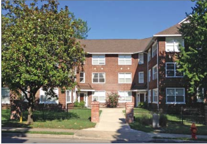
Courtyard flats providing housing choice
