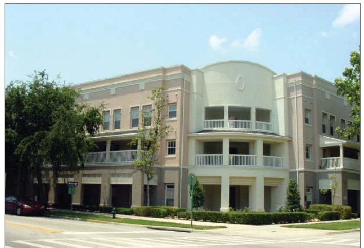
Mixed use building at a prominent intersection
