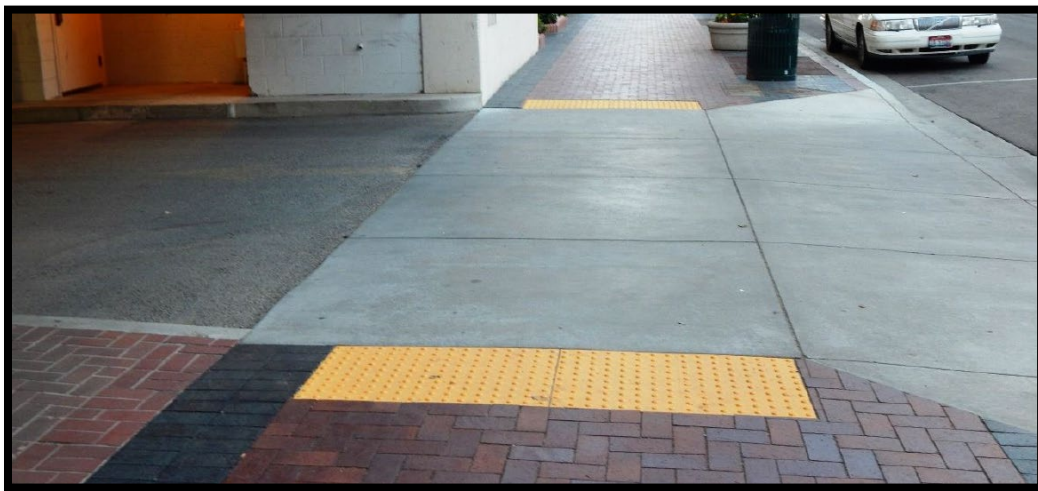
Figure 4-7: Garage Access Ramp Flush with Sidewalk
