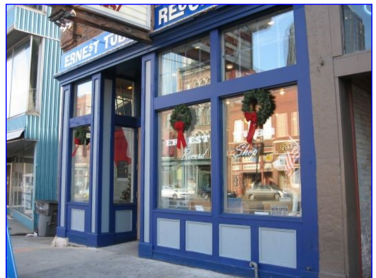
This modern storefront appropriately replicates the missing historic storefront through its incorporation of the typical storefront elements of a recessed entryway, wood-paneled bulkheads, clear glass display windows with wood frames, and clear glass transoms with wood frames. 615-880-4900
