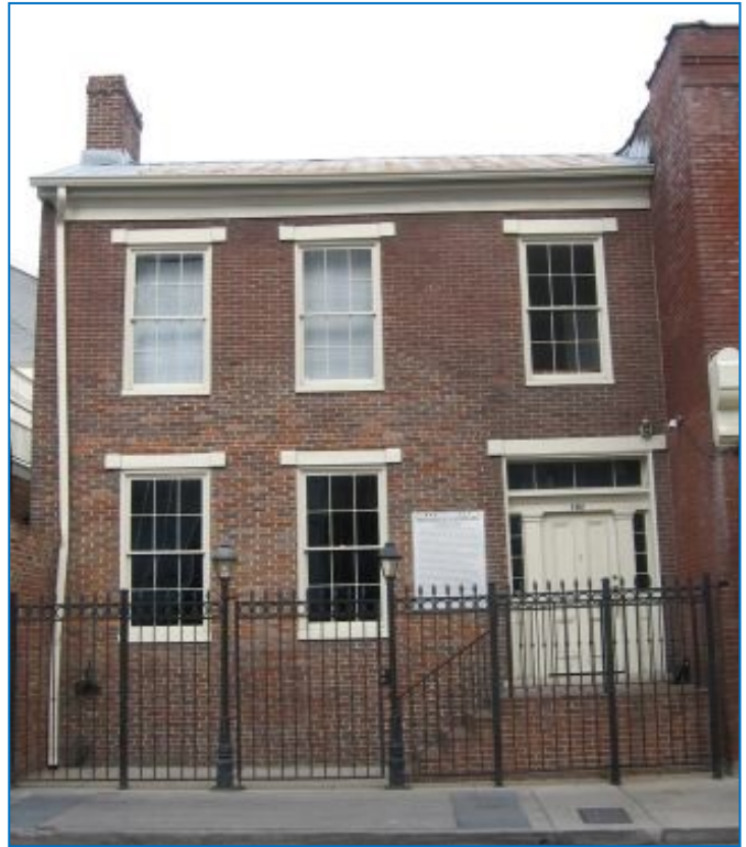
The replacement bricks and brickwork in the lower left portion of this building façade used appropriate bricks, laying pattern, joinery, tooling, and mortaring.
