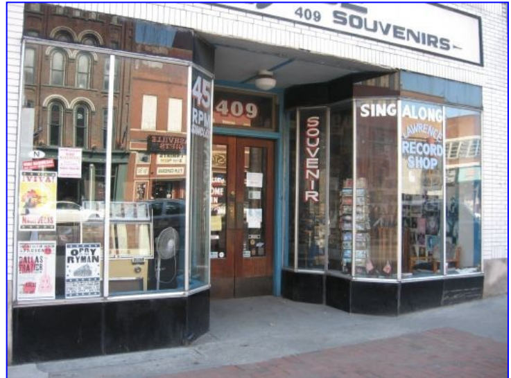
Historic storefronts such as this ca. 1930 design with Carrara glass at 409 Broadway should be retained and, if needed, repaired using materials that match the historic materials.
