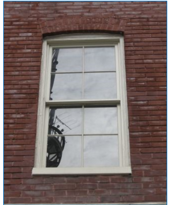
Appropriate modern four-over-four sash replacement window.
