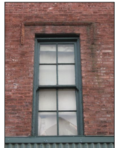
This modern replacement window is an appropriate design for this building and has a wood frame, clear glass panes, and a double-hung four-over-four configuration.
