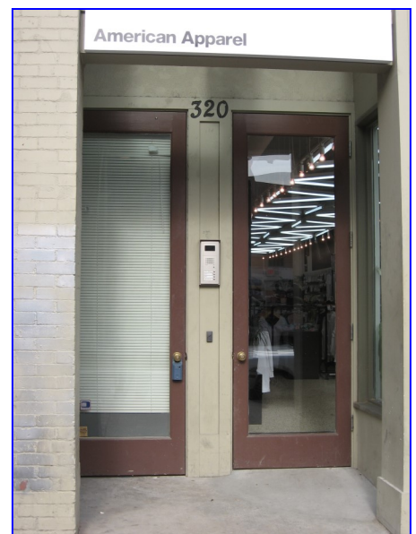
Appropriate modern doors at 320 Broadway.
