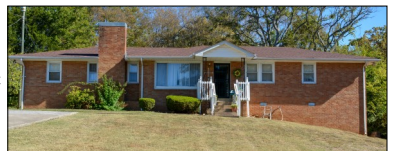
827 Youngs Lane is an example a cantilevered second level.
