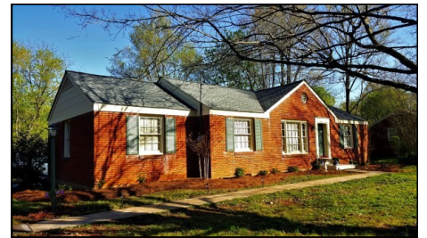
Stark-Grisham House is a spec Ranch house built by Ed Marlin from 1953-1954 on Canton Pass. Photographed by Robbie D. Jones.
