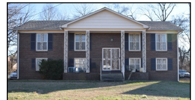
3836 Augusta Drive is an example of a two-story split level form.
