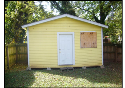
Example of a small storage building without a permanent foundation.
