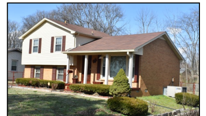
3822 Cravath Drive is an example of a one and one-half story split level form.
