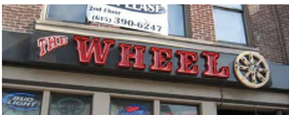
Example of raceway incorporated as sign background
