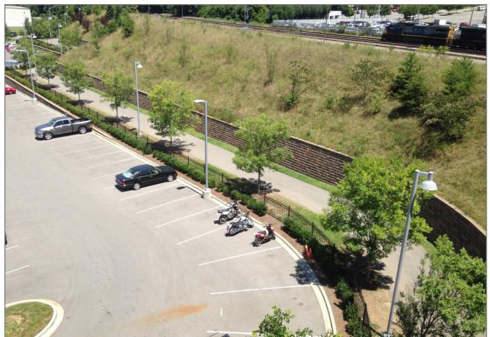
Lighting along multipurpose greenway in the Gulch
