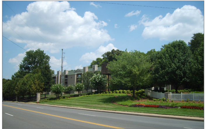
Major corridor framed by landscaping
