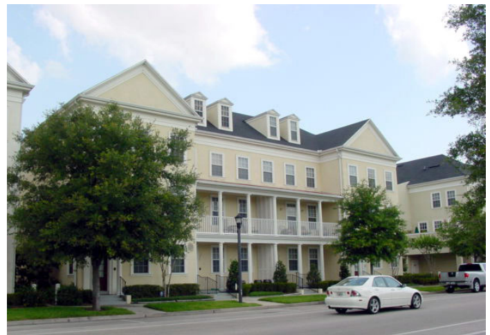
Residential building form on a mixed use corridor
