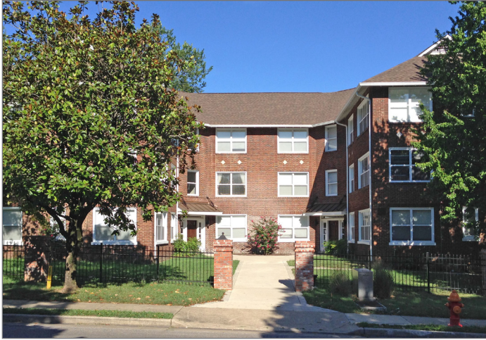
Courtyard flats providing housing choice
