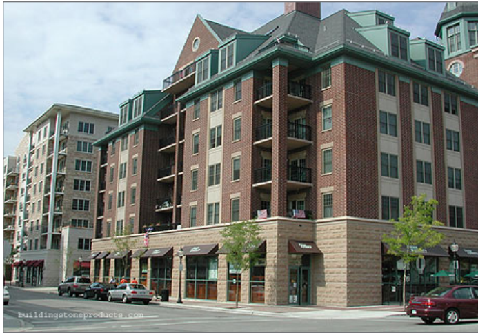
Massing and orientation of a building in T5 with distinction between the public and private realm
