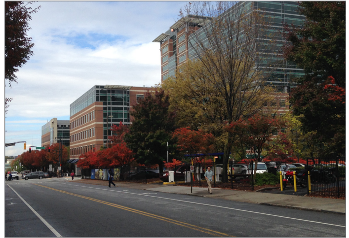
Parking located to the side and screened from the street
