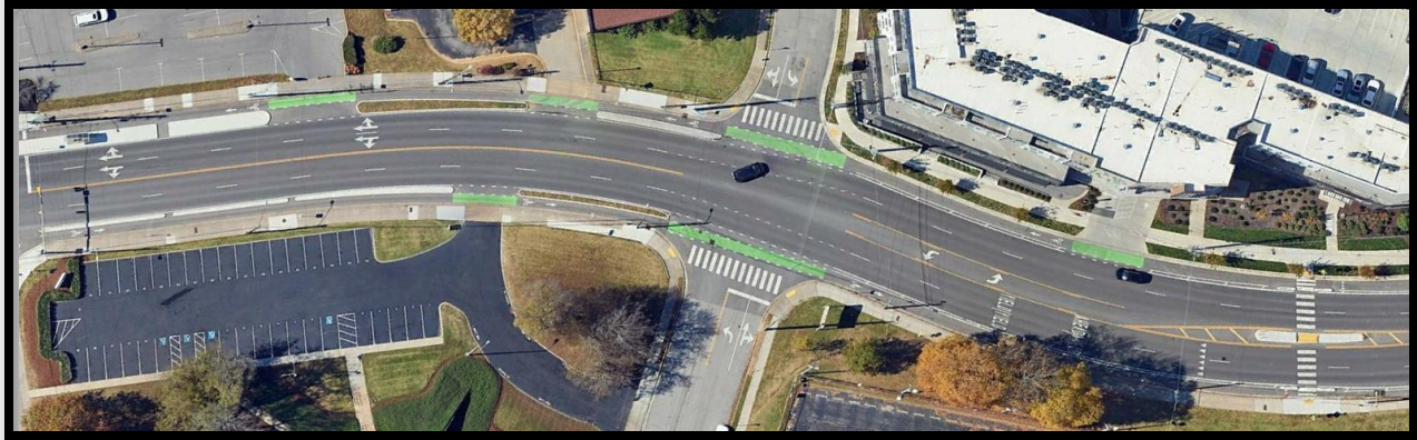
Figure 4-2: Bike Lanes on 12th Avenue South Featuring Green Pavement Markings at Driveway Crossings and Vegetative Buffers (Nashville, TN)
