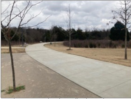
Newly constructed trail at Mill Ridge Park
