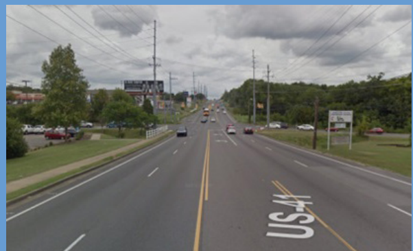
Murfreesboro Pike near Hamilton Church Road, looking north.
