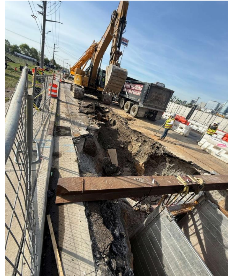
Image of Interstate Dr NES/ITS Duct Bank Installation
