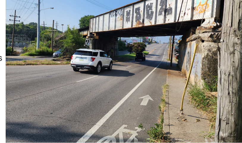
Looking southbound on Gallatin Pike at the CSX underpass.
