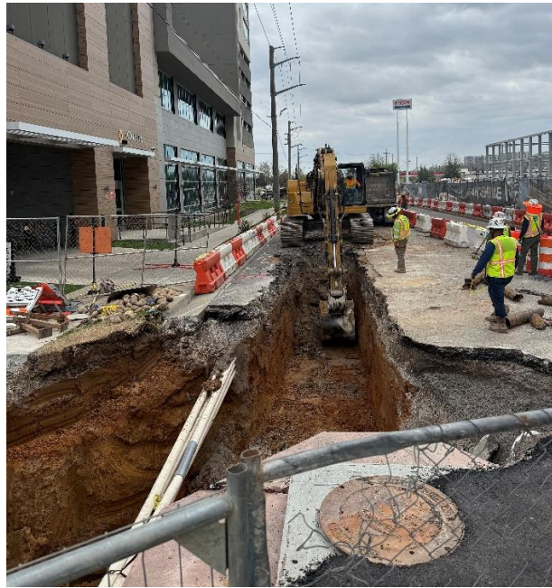
FIGURE 10: INTERSTATE DRIVE SITE PHOTO SHOWING EXCAVATION FOR THE NES/ITS DUCT BANK
