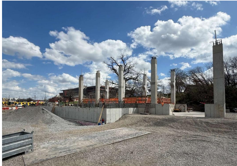
FIGURE 13: LOWER PUMP STATION SITE PHOTO
