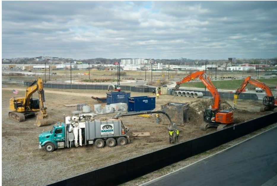
FIGURE 5: RIVER NORTH EARLY WORKS SITE PHOTO
