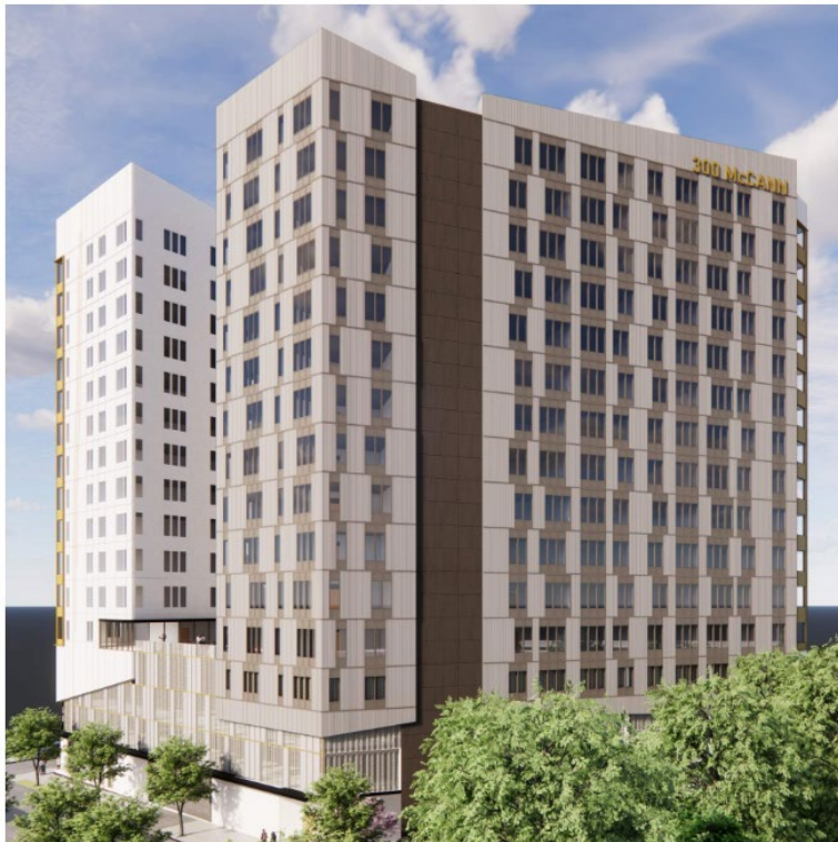
View from northeast corner
