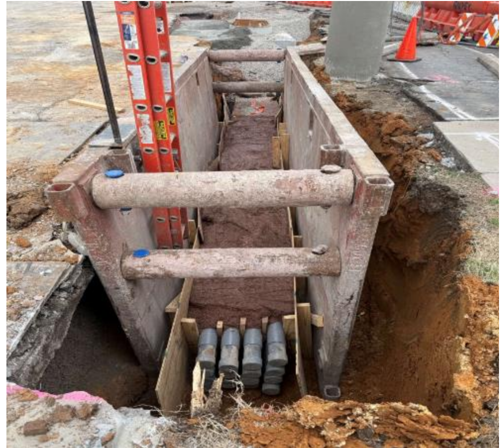
Image of Interstate Dr NES/ITS Duct Bank Installation
