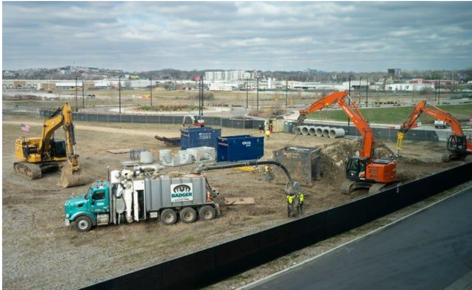
Oracle campuses early work construction
