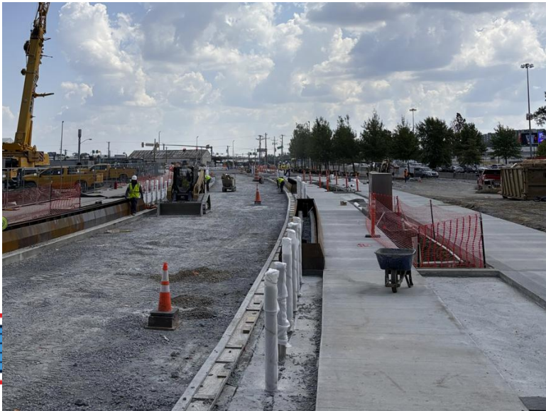
Below: Ground level looking South on S. 2 nd
