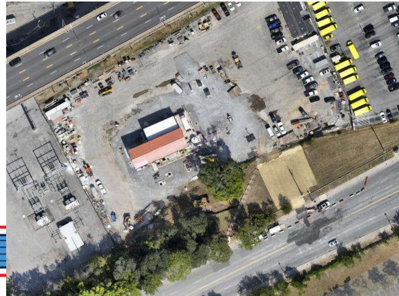
Below: Aerial Image of EB Pump Station
