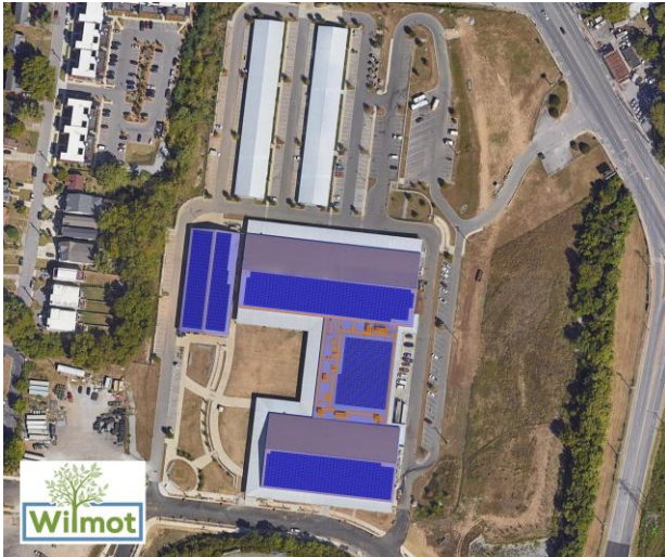
Solar array placement on Expos 1, 2, 3 and Arena
