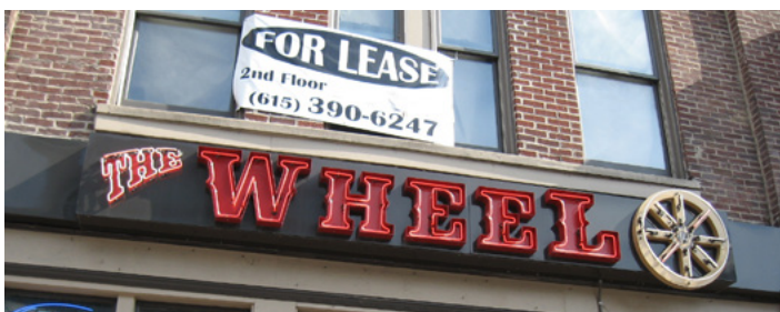
Example of raceway incorporated as sign background
