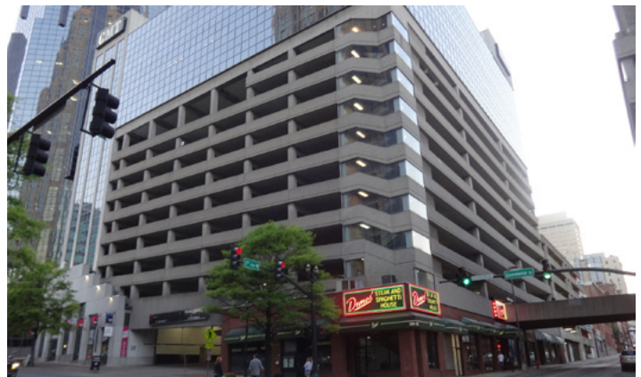
Inappropriate upper level facade treatment
